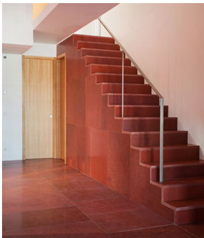
Internal paving of natural stone slabs and stairs
